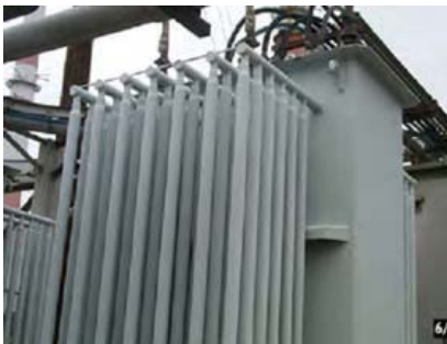
2000 kVA Transformer-Low Oil in Transformer-Reduce Transformer's capacity by square inch of cooling capacity -- Est @ 65%
